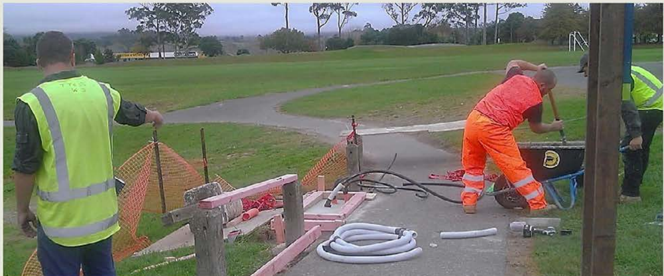
Construction continues: Construction of connecting paths is underway at McLeod Park.
